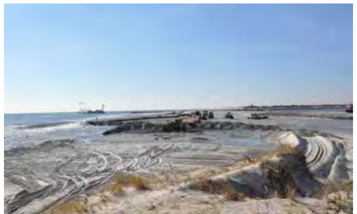
Cupsogue County Park breach closure operations are visible and nearly complete on Nov. 26, 2012, with the dredge in the background, sand pumping into the breach and earthmovers positioning the freshly pumped sand. (photo by Chris Gardner, New York District)
