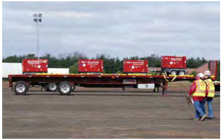
Army Corp of Engineers personnel stage and prepare generators in central New Jersey for deployment to support the Emergency Temporary Power mission in the aftermath of Hurricane Sandy. (photo by Mary Markos, St. Louis District)
